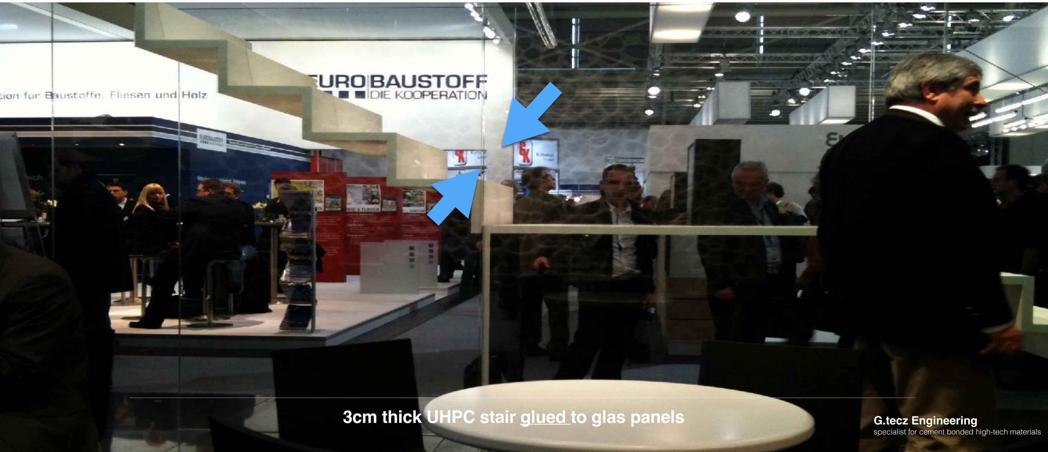
3cm thick UHPC stair glued to glas panels
